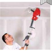
To apply tape to the ceiling, install the extension of your choice depending on the height and access. Possibility of working at heights of over 3 metres.
