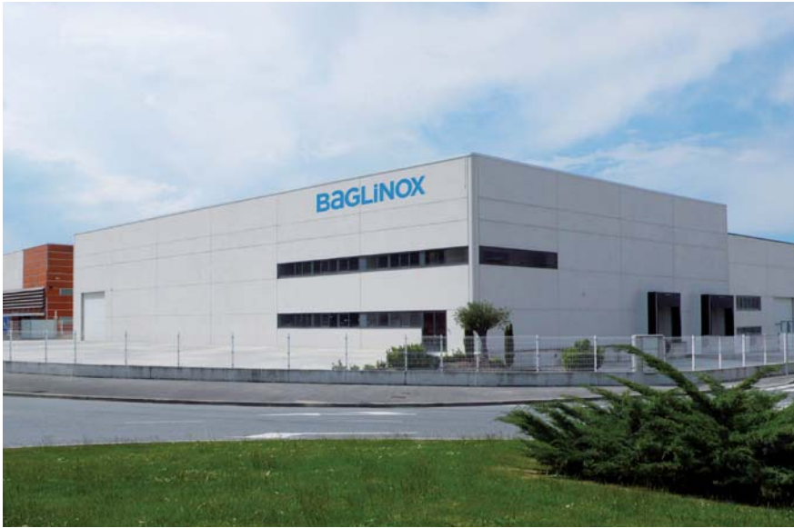
Fábrica / Factory / Usine. Orcoyen, Navarra
